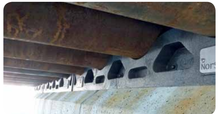
Pipe Carriers placed on concrete
