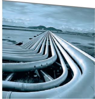
Pipelines are continuously monitored with an Omnisens system, registering small variations in temperature, strain and even vibration, to within a meter of the occurrence.
