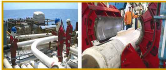
Figure 10. Injection molding polypropylene system
