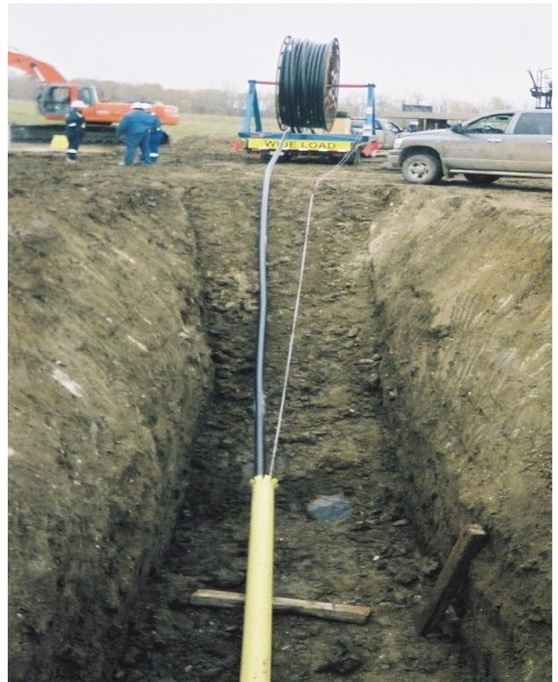
**FIGURE 4 - INSERTION AS A FREE-STANDING LINER**
