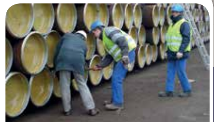
On site application of Steel Bevel Protectors and Plastic Plugs
